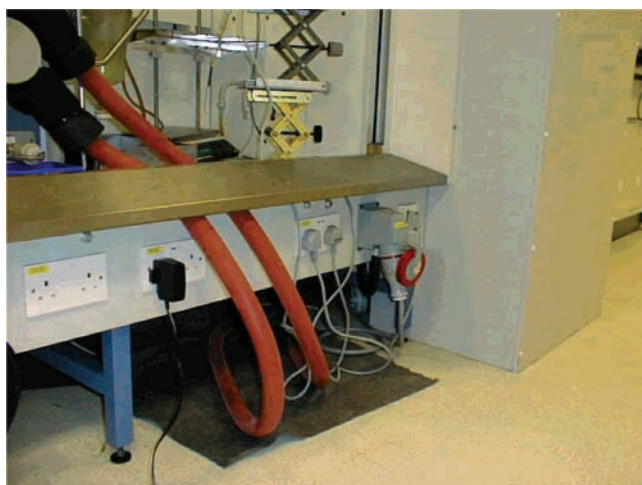
Figure 4. Picture of Huber 390 W chiller and hoses.
